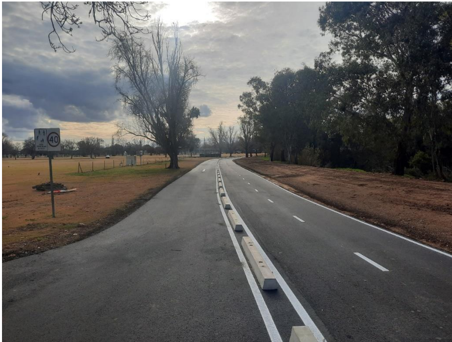
Figure 3: Example of precast castellated kerbs recently installed on the Riverside Shared Pathway in Tamworth.
